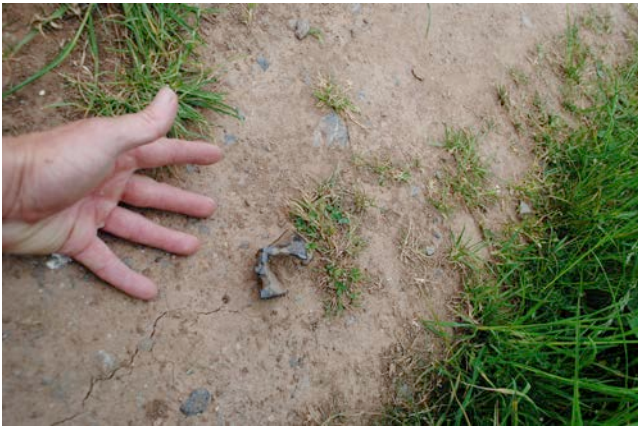
sharp metal protruding from earth trodden path
